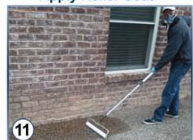
Apply Roller Coat
