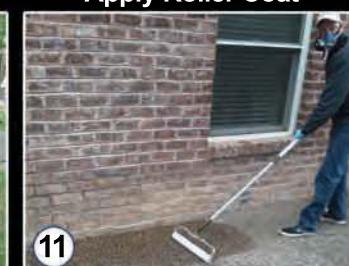
Apply Roller Coat
