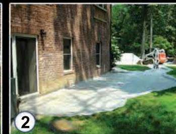
Install Geotextile Fabric
