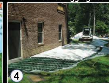
Wash Stones And Allow To Dry (Or Use Gravel-Lok Pebbles). Mix Stones With Gravel-Lok In A Cement Mixer Or Wheelbarrow
