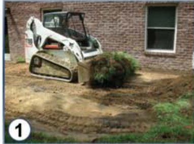
Excavate Job Site
