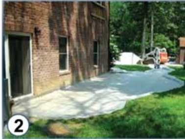
Install Geotextile Fabric
