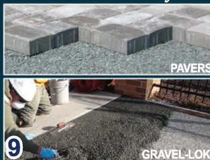
Install Surface Layer
