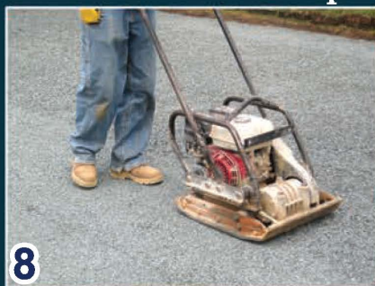
Overfill Cells & Tamp
