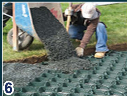
Install Surface Layer
