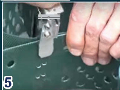
Overfill Cells & Tamp
