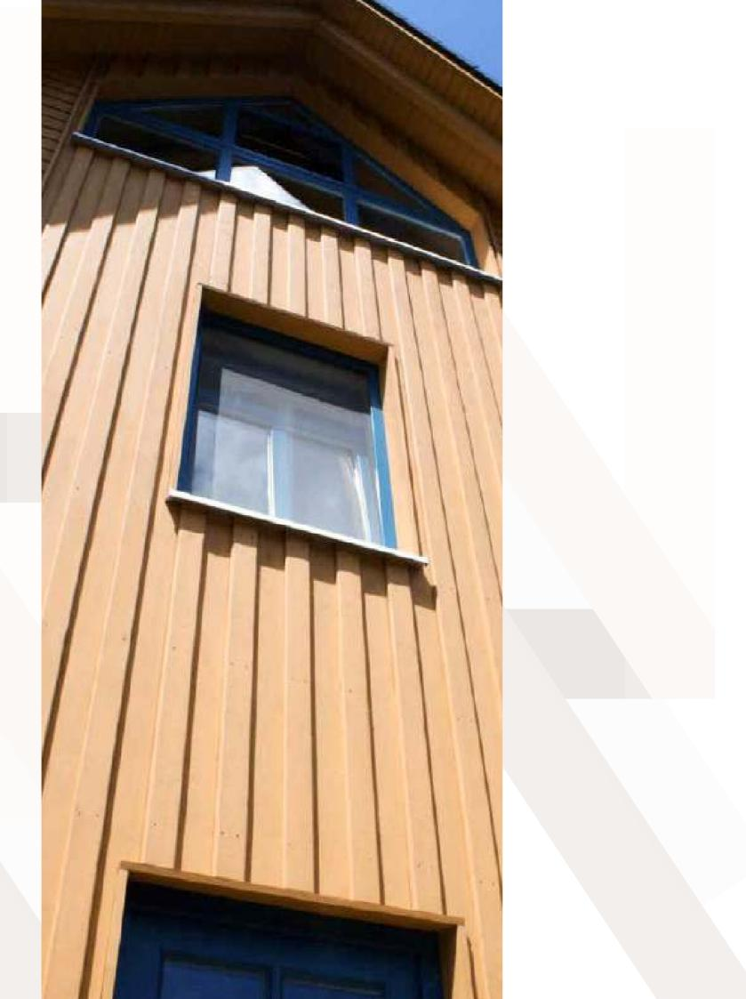
HDG's Resysta sheet and trim products are perfect for creating a classic "board and batten" siding profile to a home's exterior. While following the basic installation parameters listed below, installers have the freedom to create unique patterns and profiles to fit any home style and aesthetic desired.
