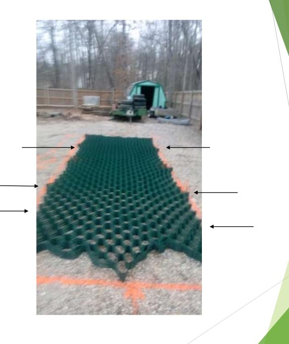
Apply the same technique to the shorter sides. First start in the middle at about the 5th cell (4 - 4.5' to the center)
