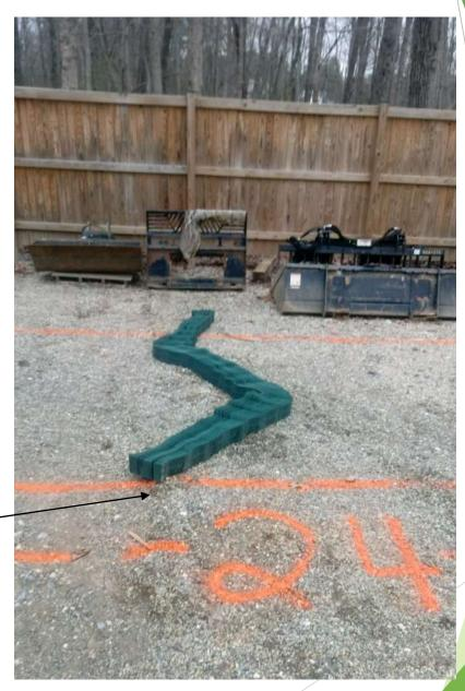
Attach the four corner cells of the grid to the four corner stakes. The grid will resemble an 'hourglass' shape.
